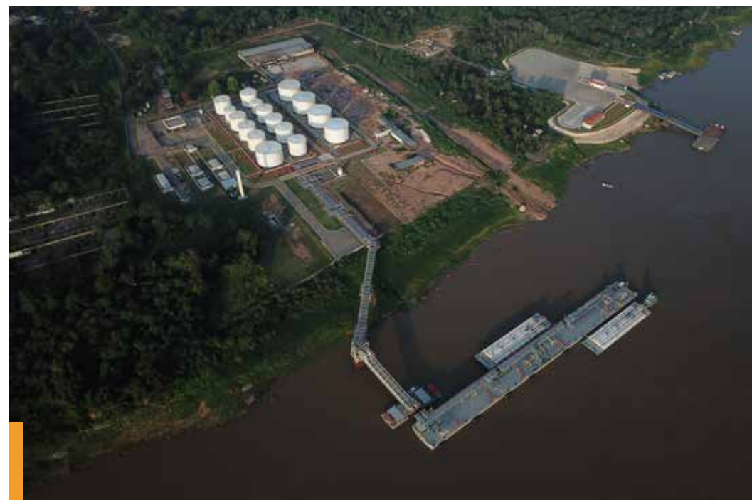
Terminal Fluvial (Itacoatiara - AM)
